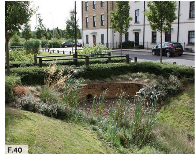
**Figure 40:** Example of swales check dam integrated with a crossing point.
